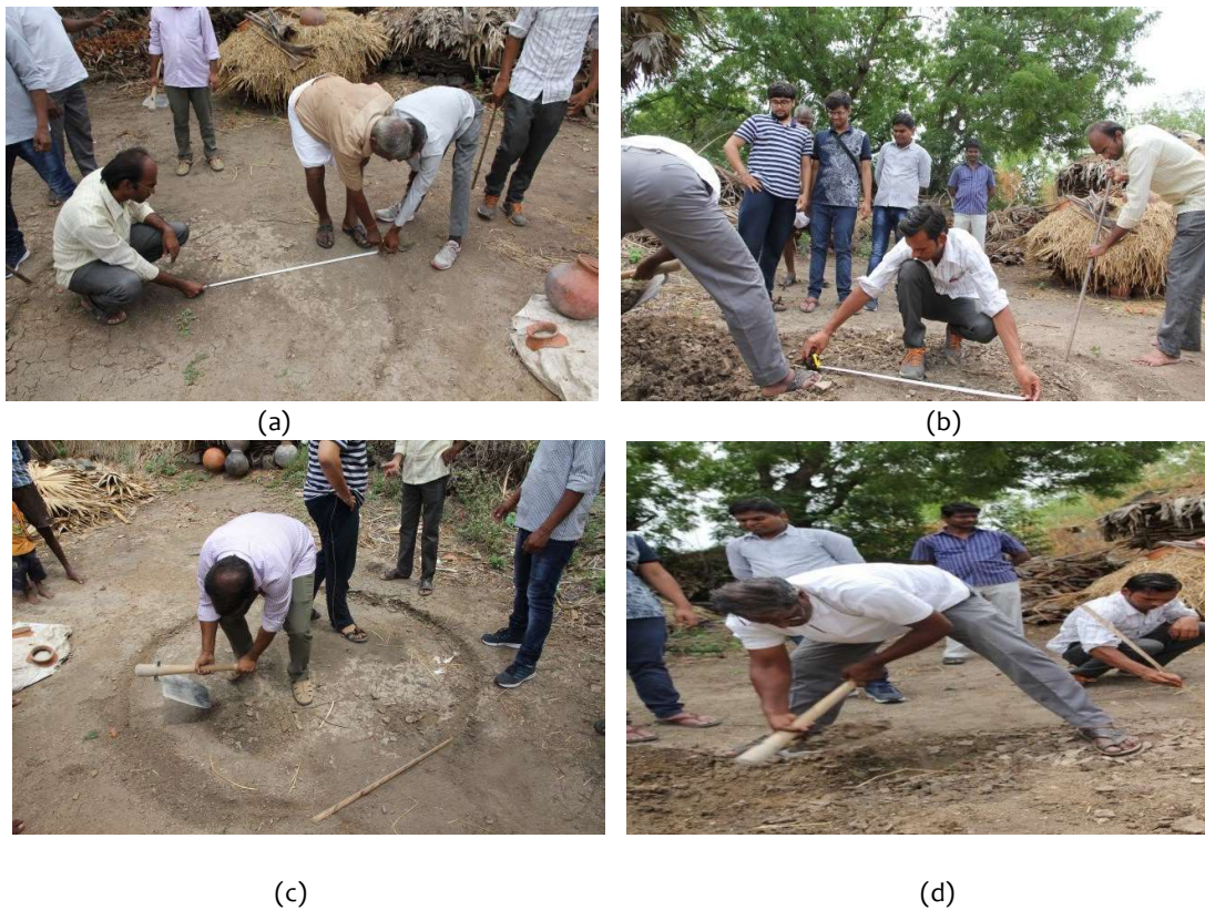
Figure 2.6: Measurements and land preparation for pottery furnace construction
