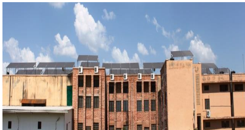
Figure 3.4 Academic Block I Building, located at “IIT, Jodhpur” Jodhpur
