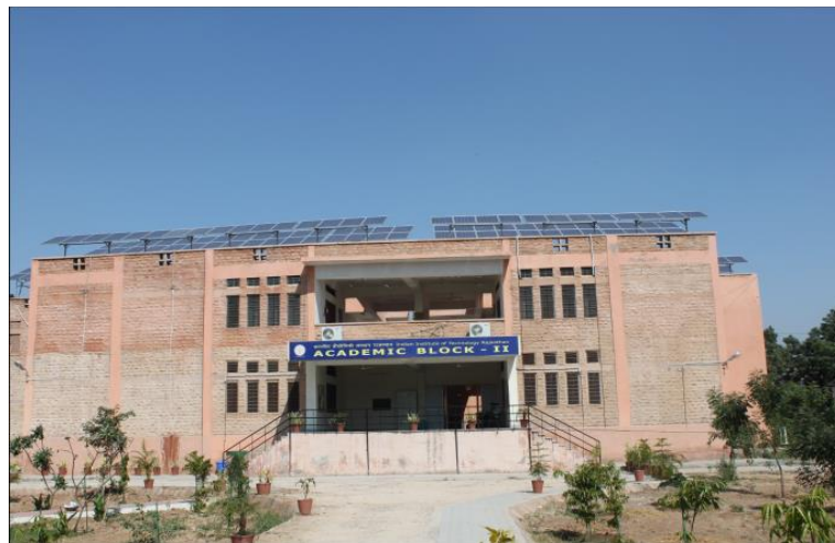
Figure 3.1 Academic block ii building, located at “IIT, jodhpur” Jodhpur
