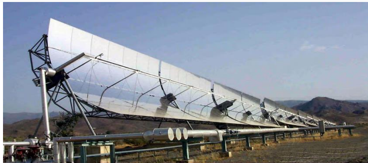
Fig 3.3: Parabolic troughs for solar collection [91]
